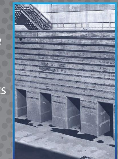
C. Gates - Gates form the upper and lower ends of the lock holding back the water and opening and closing to allow boats to pass. The lower gates of the Poe Lock are 57 feet high and weigh 225 tons each.
